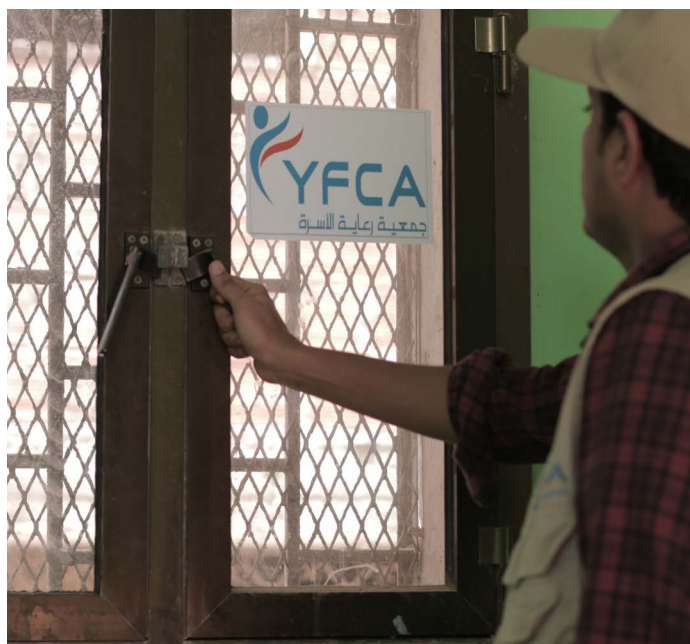
YFCA Worker repairing the window.
